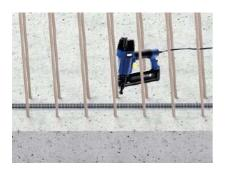
The distance between nails should not exceed 25 cm in the longitudinal direction of the swelling tape.
